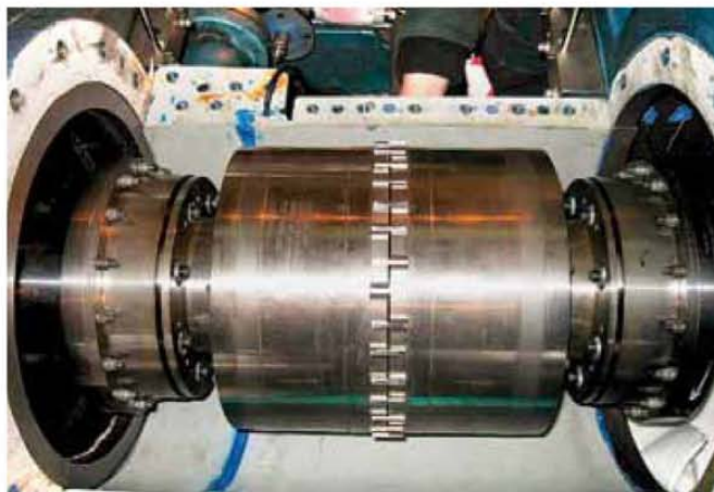
FIG. 2. Torque-meter coupling retrofit at Qenos Olefins plant.
