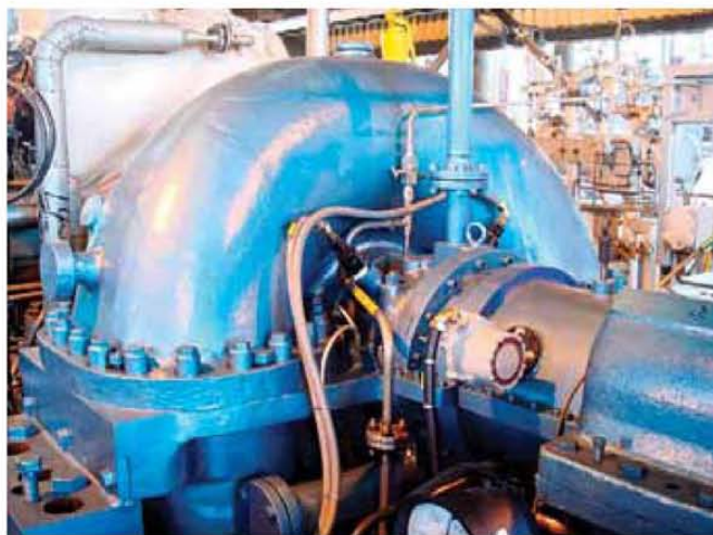
FIG. 1. Completed mechanical installation at Qenos Olefins.
